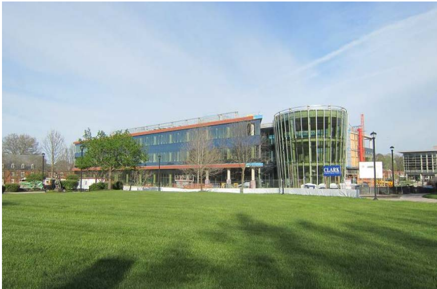
CNSMN under construction
