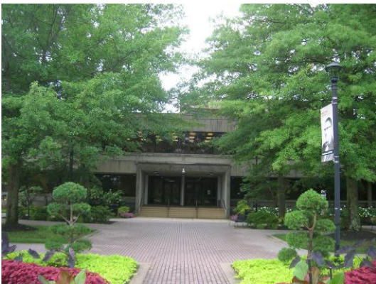
Paving area in West Courtyard
