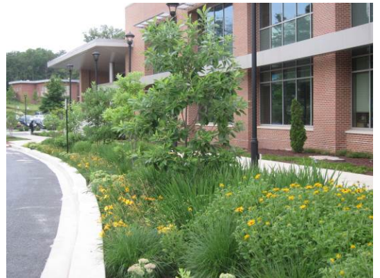
Bioretention facility near Student Center
